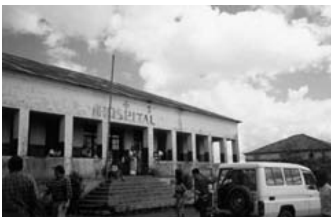
Hospital de Maniamba
